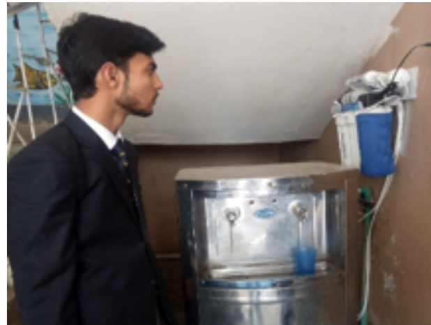
Installation of water filter at Govt Primary School, Risalpur
